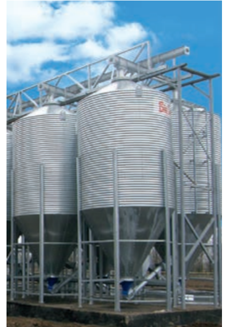
Outdoor silos for storage of ingredients
